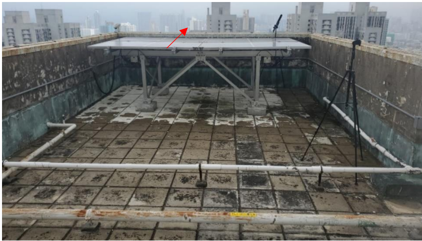
DM-4 Block 6, Tsui Chuk Garden (roof)
